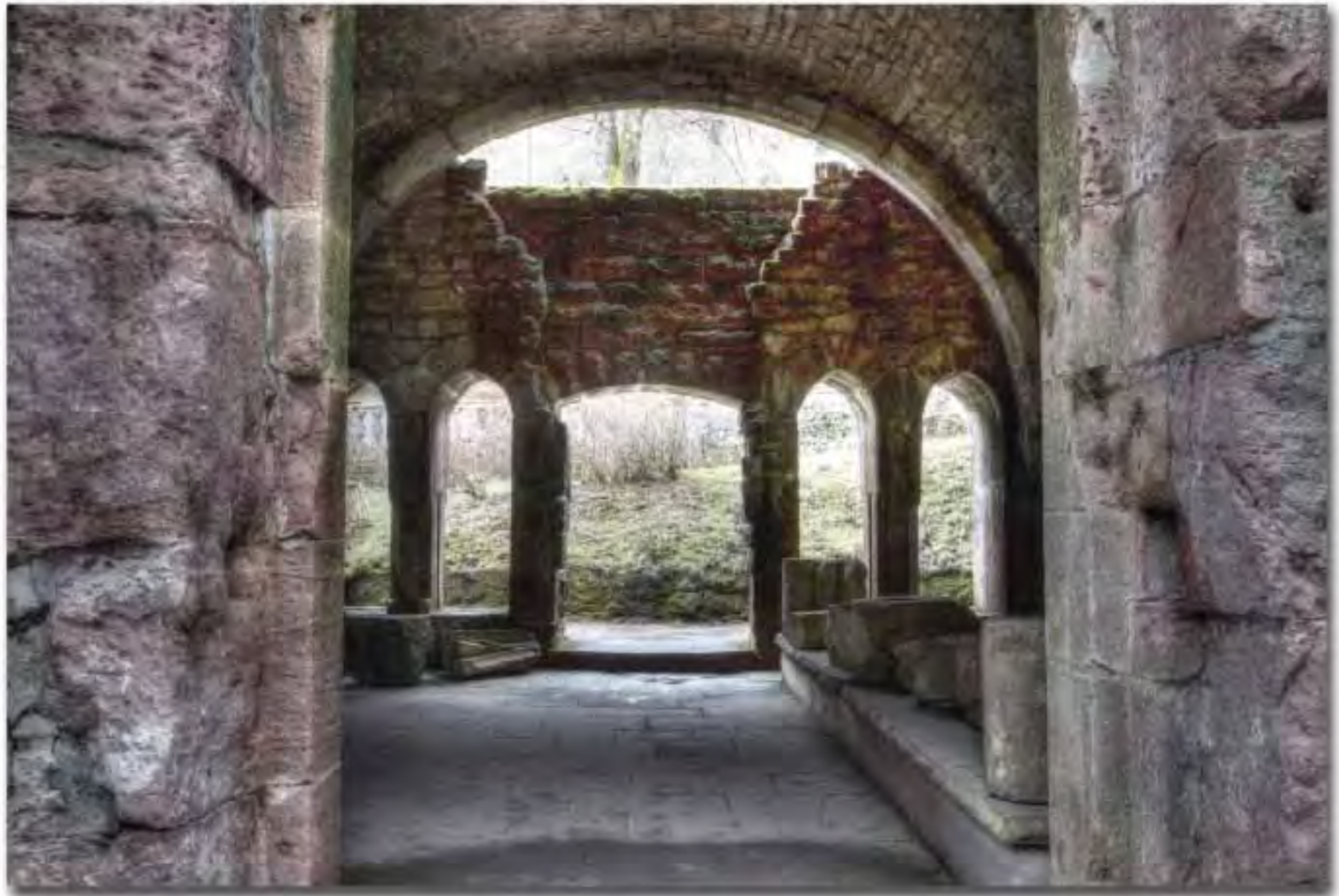
Archway of the monastery ruin of ALLERHEILIGEN in the Black Forest. Typical for many historical buildings in the region, the monastery was built out of red sandstones, which can be found in the Black Forest.
