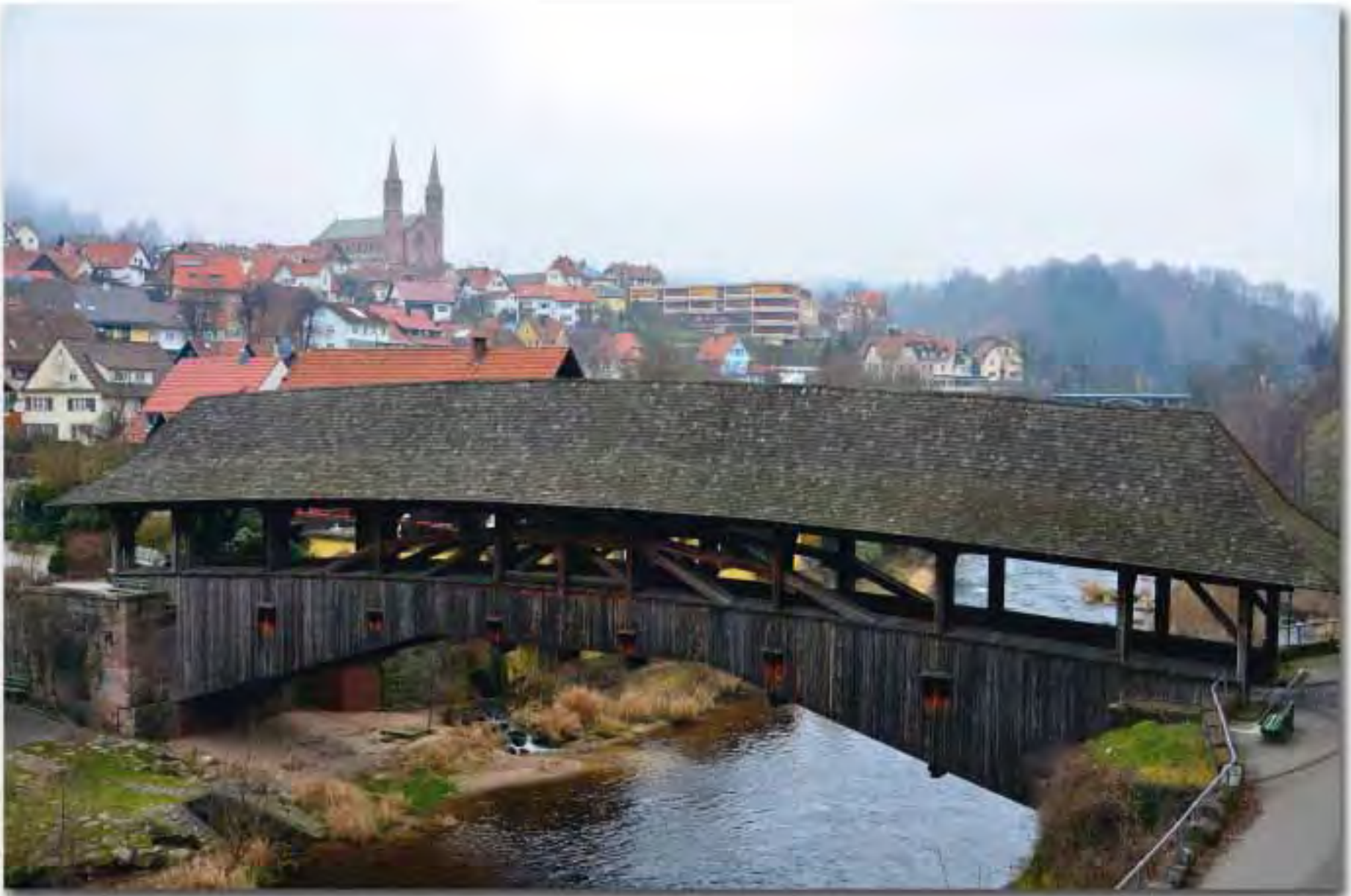
Historic bridge of the river Murg in Forbach.
