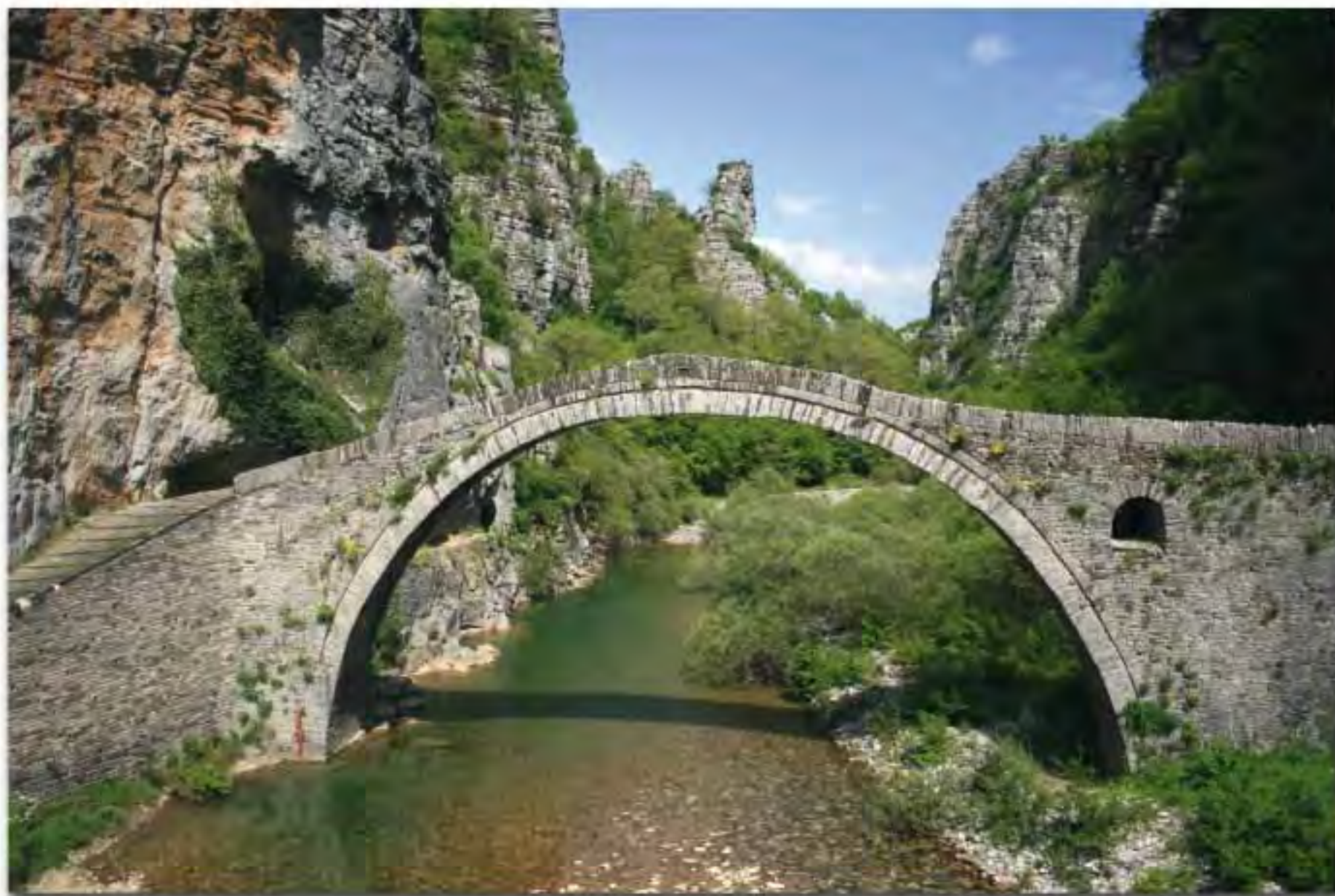
KOKKORI Arched bridge from 1750. At the river Bikaki 23,60m length and 13m height
