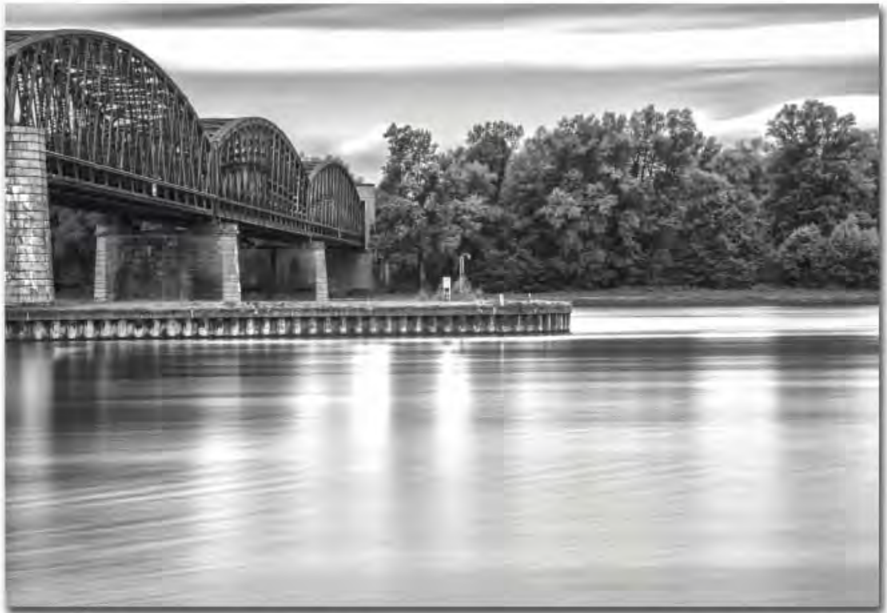
The bridge of Beinheim traversing the river Rhine. Here the Rhine is the border between Germany and France
